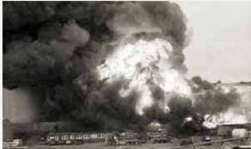
Explosion at the Vest Tank facility in Norway, following caustic washing of coker naphtha delivered by Trafigura, 24 May 2007.
