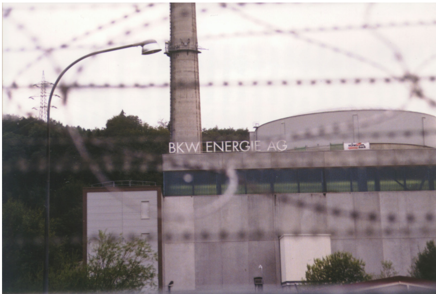
Figure 1.12 – Mühleberg nuclear power plant. Source: Fokus Antiatom
