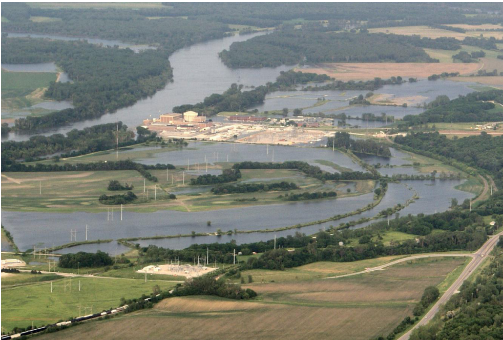
Figure 1.13 – Flooding at Fort Calhoun nuclear power plant, United States, 2011. Source: Larry Geiger, http://cryptome.org/eyeball/ne-npp-flood/ne-npp-flood.htm#Larry Geiger
