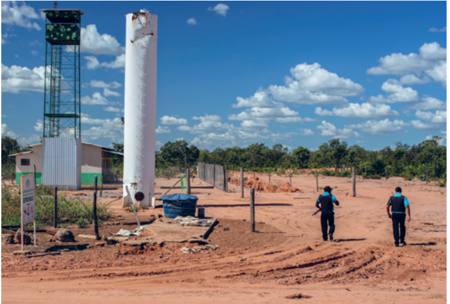
24 May 2019, Estrondo Estate, Formosa do Rio Preto: Checkpoint and watchtower manned by the Estrela Guía, private security company. ©Cruppe/Greenpeace
