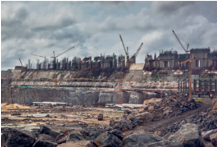
◀ 17 October 2014, Altamira, Pará: Construction of Belo Monte Dam. ©Quintanilha/Greenpeace
